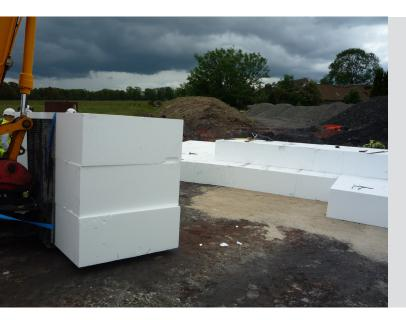
Filcor (Expanded Polystyrene) is increasingly being specified for an ever-growing range of applications. The most common applications include use as a lightweight structural fill alternative to more traditional fill materials or as a lightweight void former in structural concrete.
