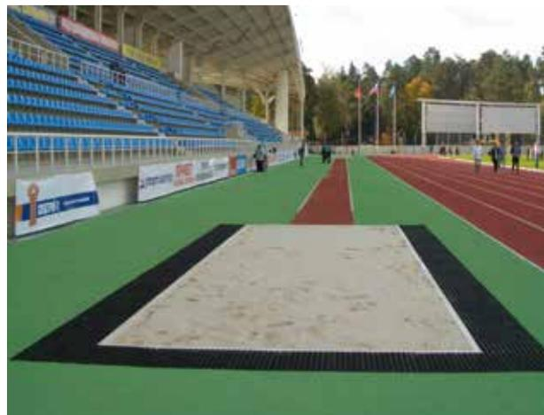
Sand pit with sand trap channels
