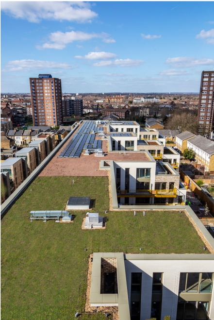
Because the development had to meet high thermal standards and provide as much amenity space to residents as possible while at the same time providing extensive attenuation - the system build ups were considerable and therefore design heights at thresholds and parapets were compromised in some areas.
