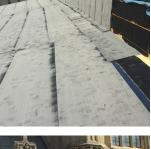
To meet the demanding brief PermaQuik PQ6100 Hot Melt Monolithic waterproofing was chosen, in combination with **MedO green roof** systems. The challenge of the shear force created by the sloping roof was solved using MedO Shear-Fix 300 and TRP140 at the eaves and centre of the roof.
