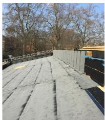
Architects Feilden+Mawson designed a timber framed building with a 300m<sup>2</sup> cold roof (insulation between the ceiling and timber cassette roof deck) with one extensive and one intensive green roof. With such a lightweight structure restraining the 15° pitch intensive green roof it required an innovative design.
