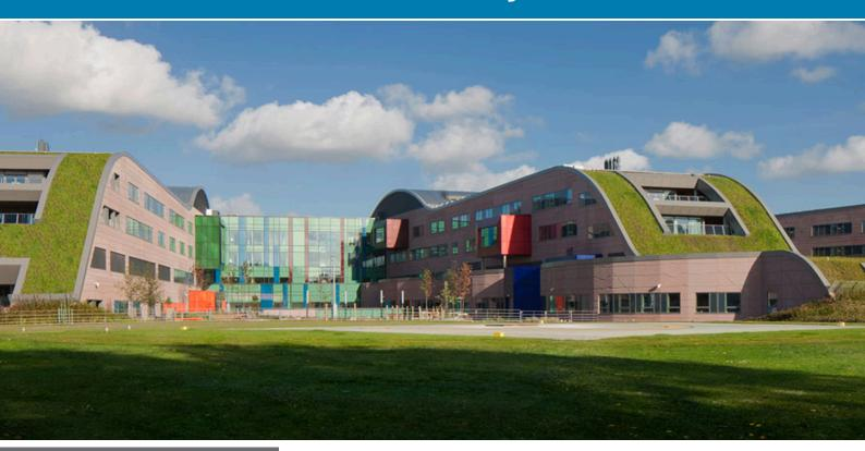
"It was important to select a waterproofing system suitable for the green roof. Radmat **Building Products** selected a two coat Liquid Applied Membrane chosen for its speed of installation and elastomeric properties allowing it to expand and contract with the building. The ease of application also meant a safer process for those working on the less accessible areas of the roof."
