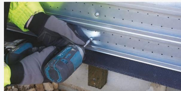
1 SureBrick can be fixed to many different backing wall types, including SFS, timber frame or concrete.
