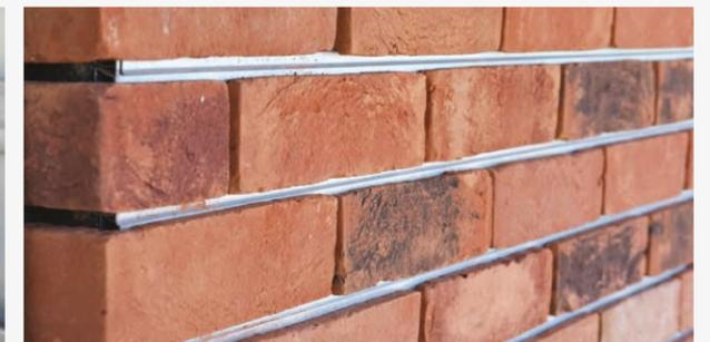
3 Specially profiled bricks are then simply clipped or slid into place before finishing with pointing mortar.
