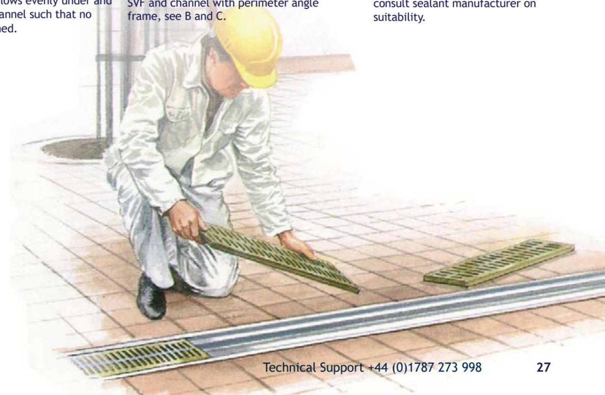
**B. Drainage Channel profile SVF - for use with vinyl and other flexible sheet material**
