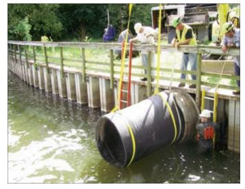
48" CheckMate<sup>®</sup> installed in a storm sewer drain to stop backflow from flooding a residential area.
