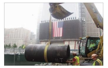
48" CheckMate<sup>®</sup> installed at the Freedom Tower for stormwater drainage.
