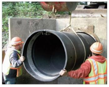
48" CheckMate<sup>®</sup> Valve replacing a faulty flapgate in a CSO application.
