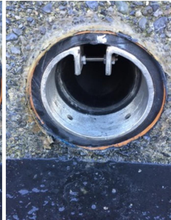
Insert CheckMate fully into pipe
