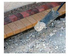
Step 2 Lay a bed of concrete to the correct level.
