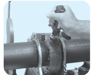
8. Check that the pipe ends are matching. If not correct either by re-clamp the pipe (alignment) and/or repeat trimming. After re-clamping it is necessary to trim the pipe-end again with a planer.
