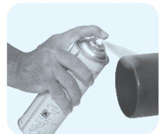
4. Apply silicone lubricant on the rubber seal and sparsely on the spigot end
