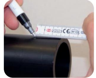
4. Measure the area which must be peeled with a measuring tape on the pipe and mark with a permanent marker.
