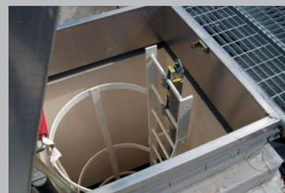
Above the 915 mm x 760 mm S-50T roof access hatch, with its LadderUP Safety Post below, which will provide a secondary means of escape from the flat roof area
