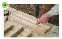
Starting from the centre mark the position of the spindles on the handrail. For easier fitting start the screws in position on the rail before attaching the spindles.
