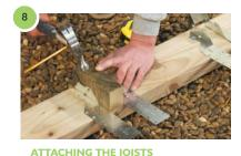
After marking the position of the joists at 400mm centres on the side beams, attach the joist hangers with galvanised nails. Use an offcut from a joist as a guide.
