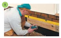
After cutting to length attach the ledger to the wall with suitable bolts. A I Omm gap should be spaced between the wall and the ledger to ensure drainage.
