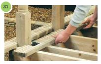
When notching the boards leave a 2 - 3mm gap around the post to allow for movement of the boards.
