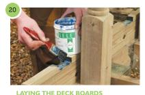
After carefully marking the boards notch out positions for the posts and treat with End-
