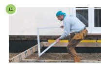
Check the beams are square using a 3, 4, 5 square, reinforcing all the corners using a framing anchor.
