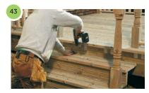
Starting from the bottom fix the boards by screwing through the face into the stair stringers.
