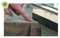
Cut the end of the top rail at a 45 degree mitre (for a 90 degree join) and fix using screws or deck rail ties.
