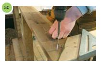
Cut the next piece of handrail at 45 degrees, butt to the original piece and fix using screws or deck rail ties.
