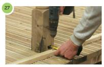
Once all the boards are fixed, determine the position of the edge of the deck. Attach a baton as a temporary guide line.
