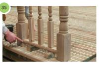
Use supports to help ensure the rail is level. Make sure there is sufficient space to fit the bottom angle brackets. Ensure the gap between the deck board and base rail is no greater than 100mm.
