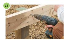
Attach the posts to the beams using coach bolts or landscape screws.
