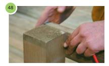
Ensuring the back rail is square with the newel post fix using two or more galvanised or stainless steel screws.
