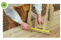
Use a spacer to ensure that the spindles are evenly spread. The maximum gap between the spindles must be no more than 100mm.
