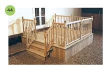
The finished deck fitted with the Arbordeck classic handrail. The sides of our deck have been cloaked with deck boards. Adequate ventilation has been provided to allow the substructure to dry after rain.
