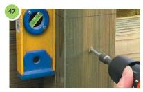
Holding the post vertical and with your mark at deck level, attach the post using the landscape screws.
