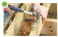
For aesthetic benefit our deck boards are fixed with deck clips. Nail the deck clips to the leading edge of the board. Space the deck clips about 50mm from each joist. Using suitable deck screws is also a good way of fixing your deck. Fix your screws 25% in from each side of the boards and use two screws per board, per joist.
