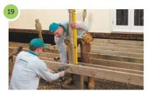
Ensure the newel post is vertical and attach it to the inside of the beams with landscape screws or coach bolts. Repeat this process around the inside perimeter of the deck, spacing the posts at a maximum of 1800mm centres.
