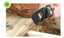
Skew screw through the side of the deck board to attach the board to each joist. If necessary pre-drill at the ends of the boards to prevent splitting.
