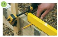
Adjust the height of the side beams to allow a slight fall in the deck away from the house. This will ensure the deck drains correctly.
