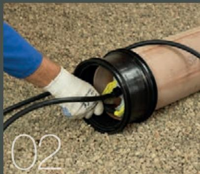
02 Fit expanding stoppers in the end of all pipelines and branches
