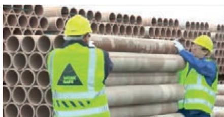
For the top row: Lift down the pipe from the outside of the top row of the pipe pack.
