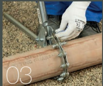
03 Hook the chain onto the jaw of the pipe cutter
