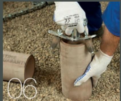
06 Remove any sharp edges with pipe trimmer
