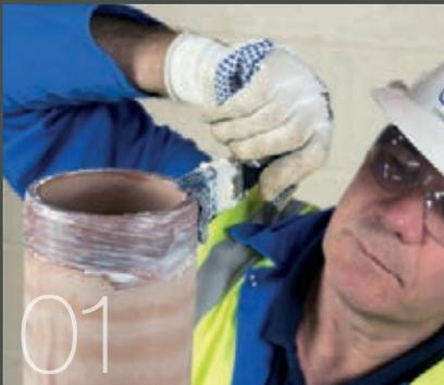
01 Lubricate the pipe end
