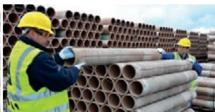
Working inwards to maintain pack stability, slide the next three pipes out parallel and lift down.
