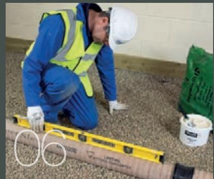
06 Check the pipeline is laid to the correct gradient
