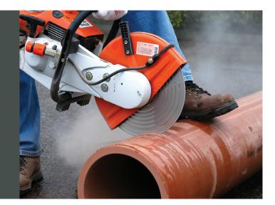
This guide will help you to improve your pipe cutting technique according to the pipe diameter you are using. Appropriate selection will make installation quicker and easier on site. Unnecessary pipe cutting can be avoided by the use of standard short length pipes at 0.3, 0.6 and 1.0m. These can be used to adjust the pipeline length at manhole and junction positions. Where cutting is necessary, chain cutters, diamond tipped and carborundum masonry saw blades can be used as advised below.
