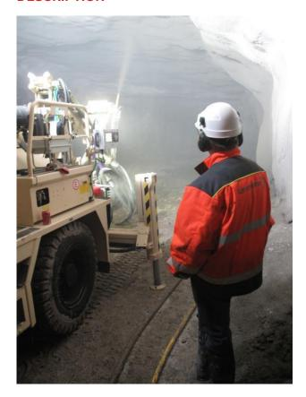
TamShot 80AF is commonly used for wet mix shotcrete processes in the tunnelling and mining industry. The product is applied where initial rock support is needed or where a permanent lining has been designed (single shell tunnel lining).
